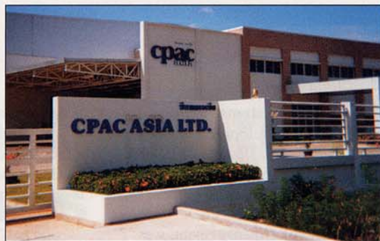
The newest CPAC Imaging chemical manufacturing plant, near Bangkok, Thailand, was established in 1999.
